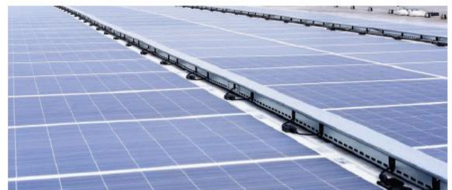
Lightweight modules on polymer membrane roof.
