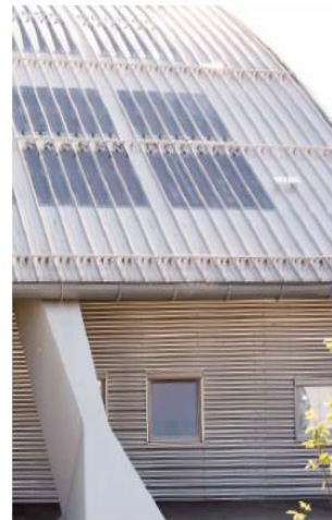
Flexible modules on aluminium roof.
